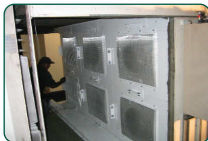
19,000 cfm at 6.5" TSP with built-in redundancy to ensure up time
