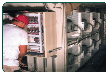
Factory-engineered controls decrease installation time and improve reliability
