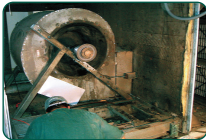
Hospital retrofit example completed in 8 hours
