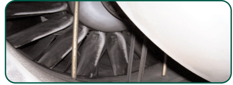
Rising Maintenance Costs and Increasing Downtime
